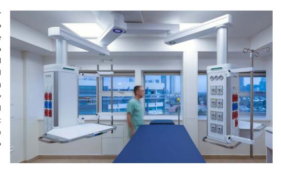
With our unique solution, equipment can be mounted from various sides of the Boom/Pendant ensuring optimal accessibility to the equipment and patient.
